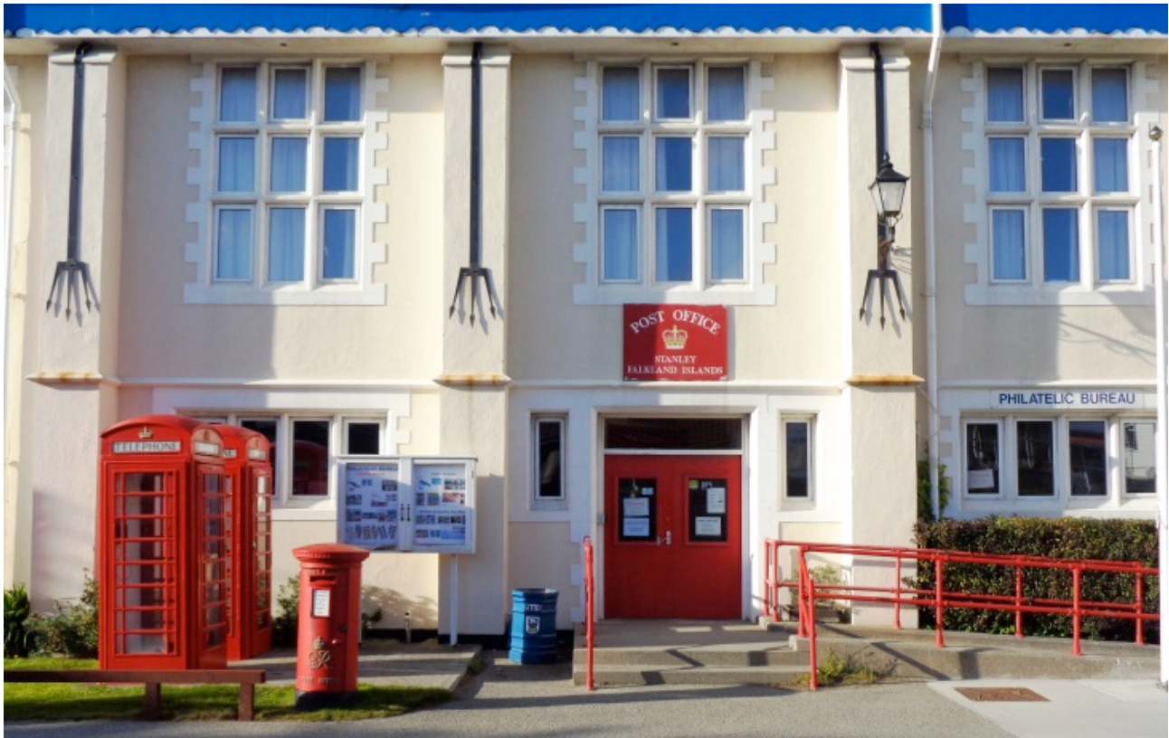
Figure 9: Stanley Post Office
