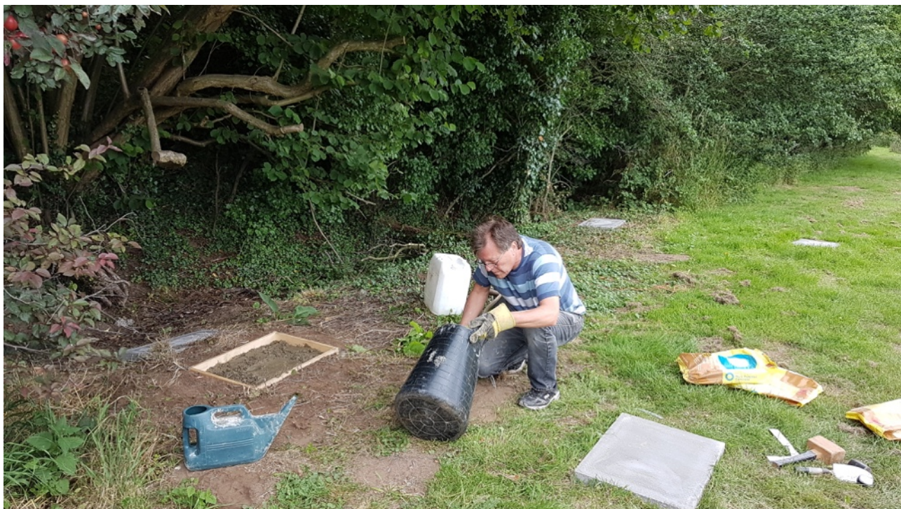
Mike Whybray mixing concrete for the laying of the first slab.
