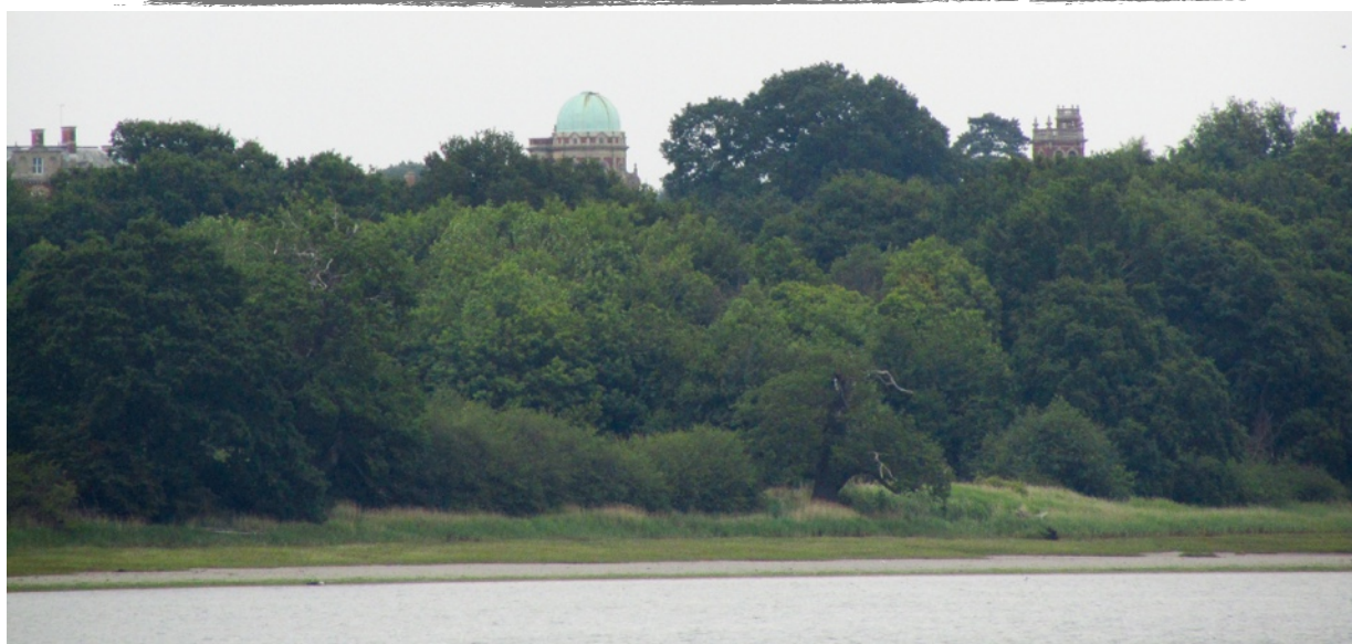
Orwell Park School Observatory and clock tower from the River Orwell
